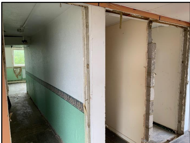
Soft Strip in Progress
