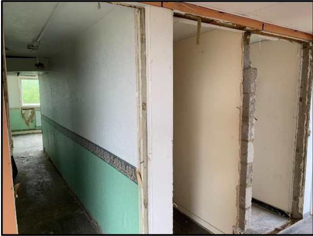
Soft Strip in Progress
