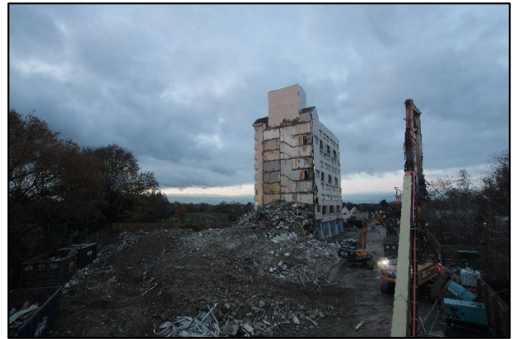
Cladding Removed to Remaining Structure
