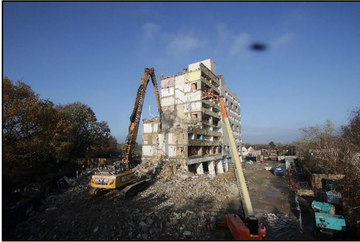
Zone 3 In Progress
