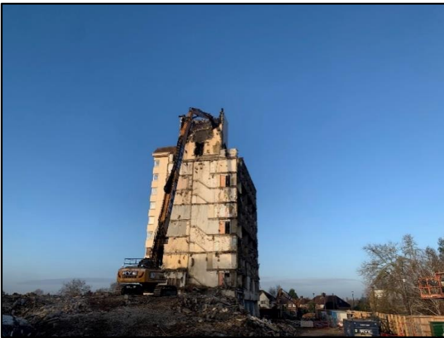
Water Tank Room And Lift Overrun In Progress
