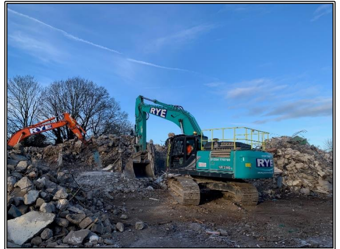
Excavators moving material and breaking a slab
