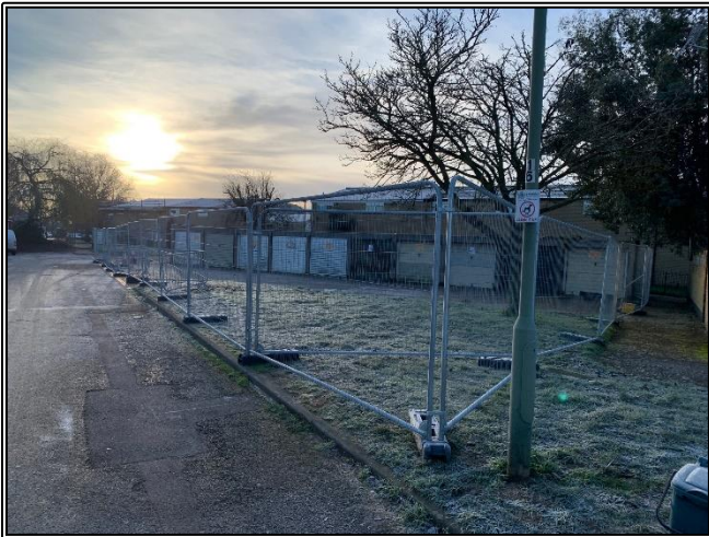
Fencing around the garages
