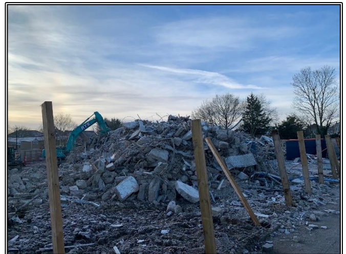
Felix Road hoarding in progress
