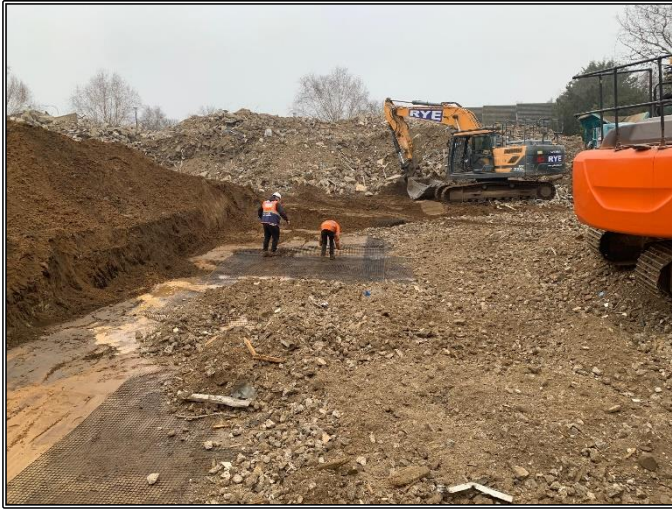
Reduced Dig and Preparing to Crush Concrete
