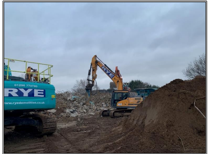
Breaking up Large Pieces of Concrete
