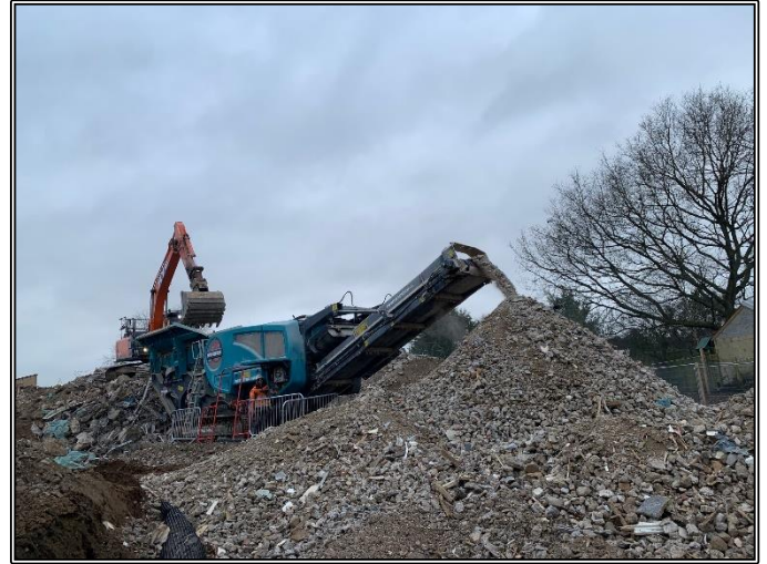
Crushing Large Pieces of Concrete
