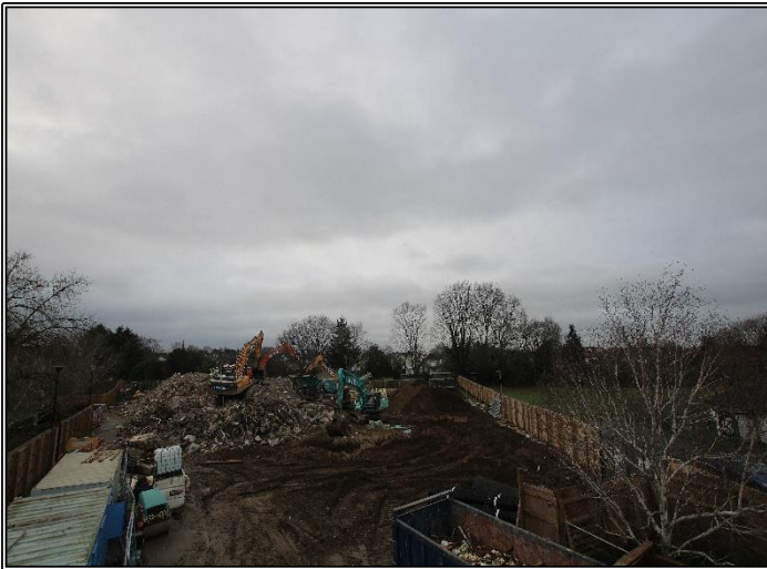
Overview of Site
