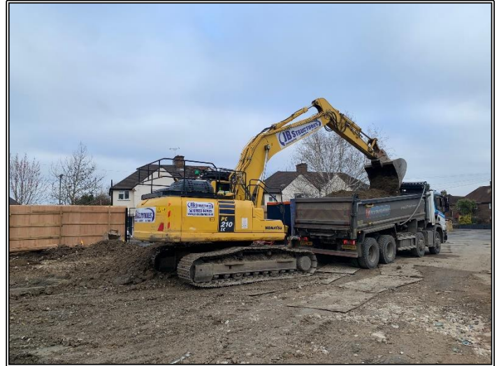
Section of Completed Piling Mat
