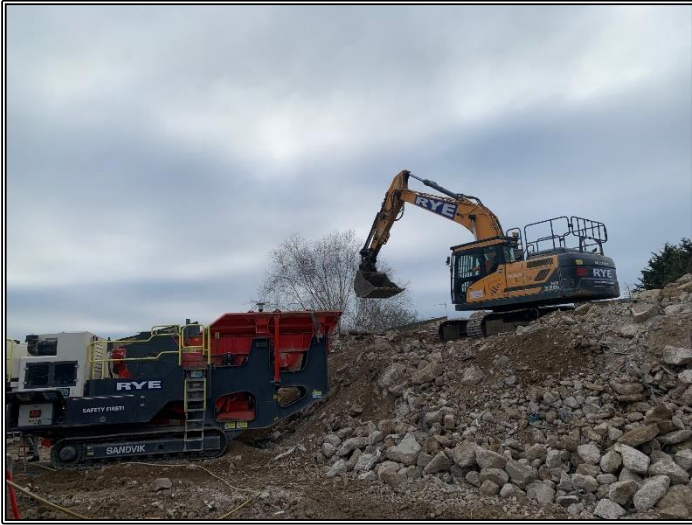
Piling Mat Works in Progress
