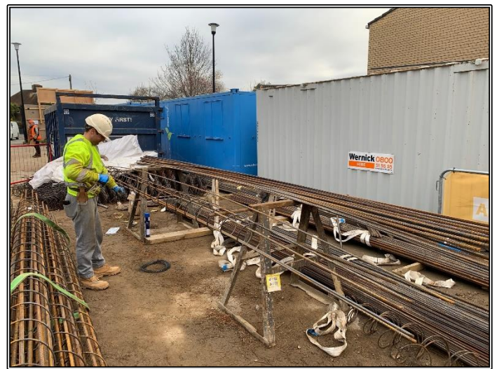
Fixing Steel Cages
