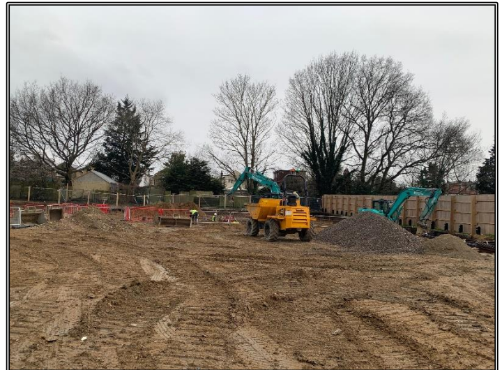
Overview Of Site
