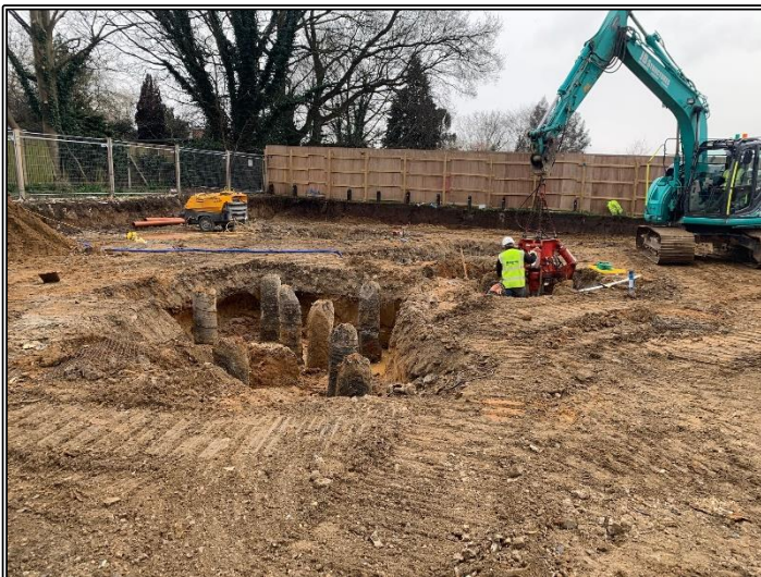
Trimming Piles
