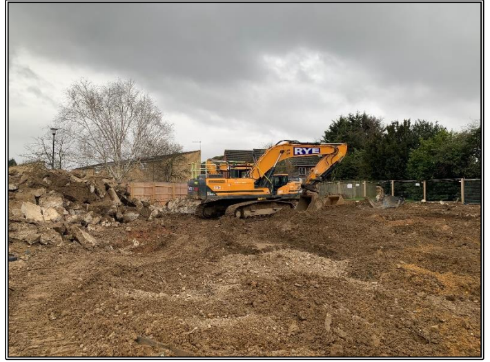
Final Existing Foundation Removed
