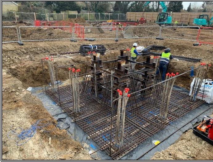
Tower Crane Base In Progress
