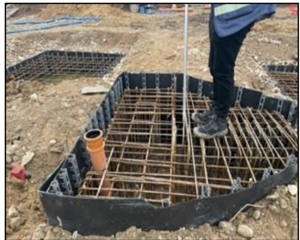
Pile caps and drainage
