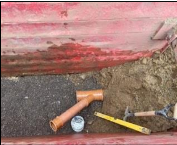
Drainage being installed
