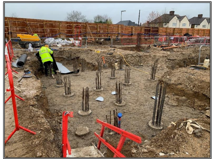
Stair Core Pile Caps
