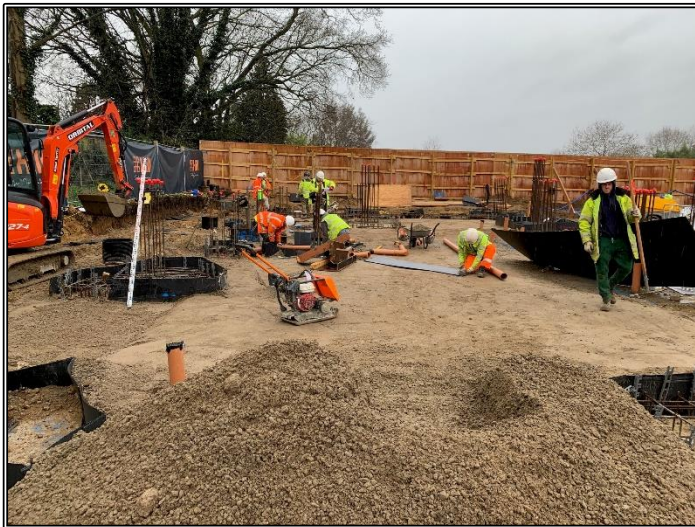
Ground Floor Blinding
