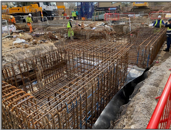
Lift Shaft & Stair Core Reinforcement
