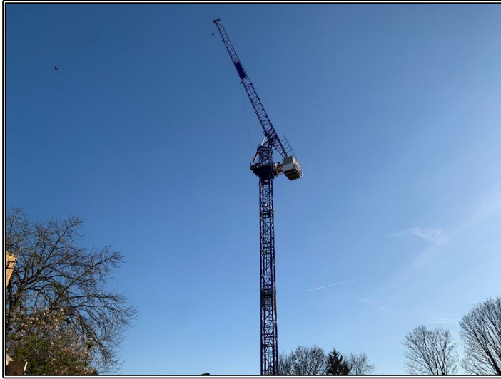
Tower Crane Complete
