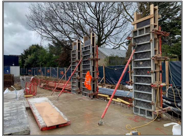
Preparing Ground Floor Columns
