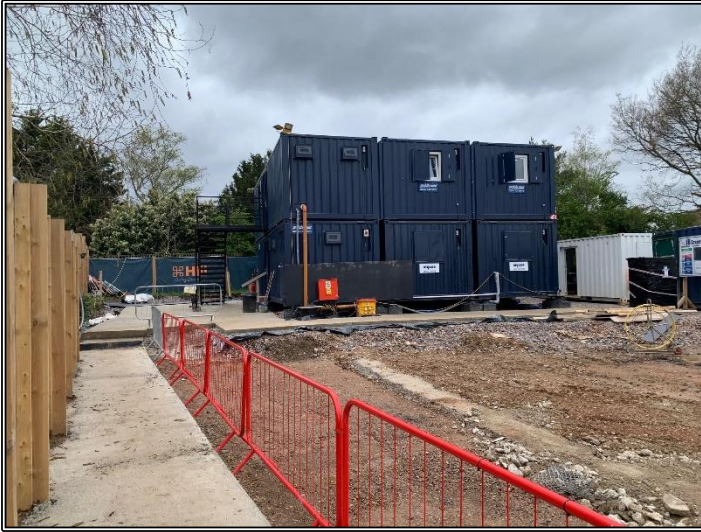
New Site Offices
