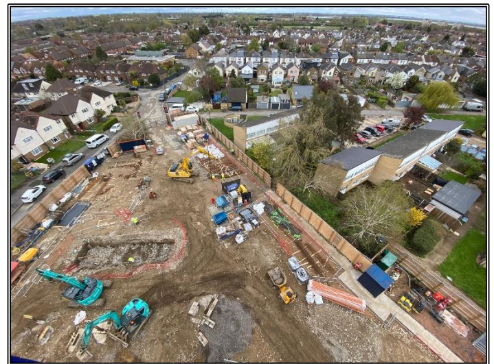
Aerial view to Front of Site
