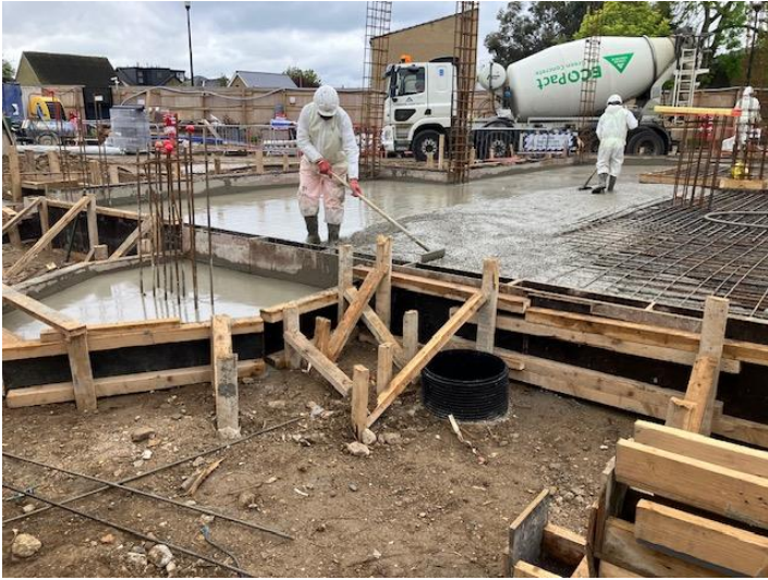
Pouring final section of Ground floor slab
