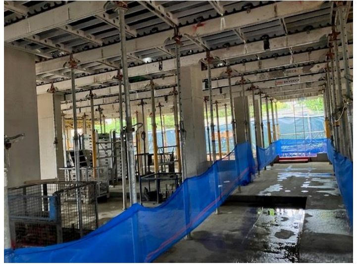
Ground floor slab with decking to First floor erected
