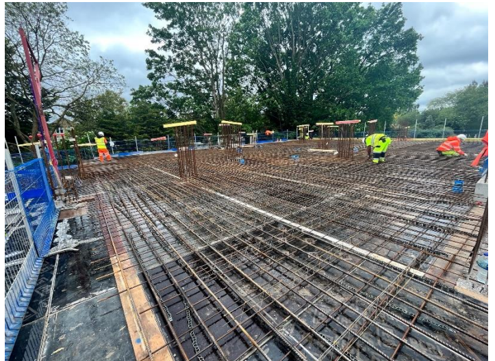
1 st floor slab reinforcement
