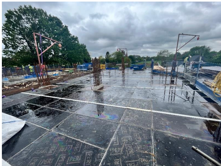
1 st floor decking
