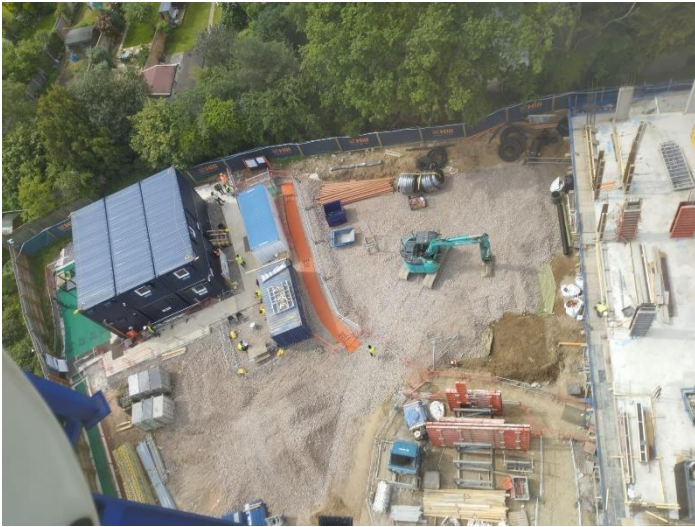
Overview of Site Compound
