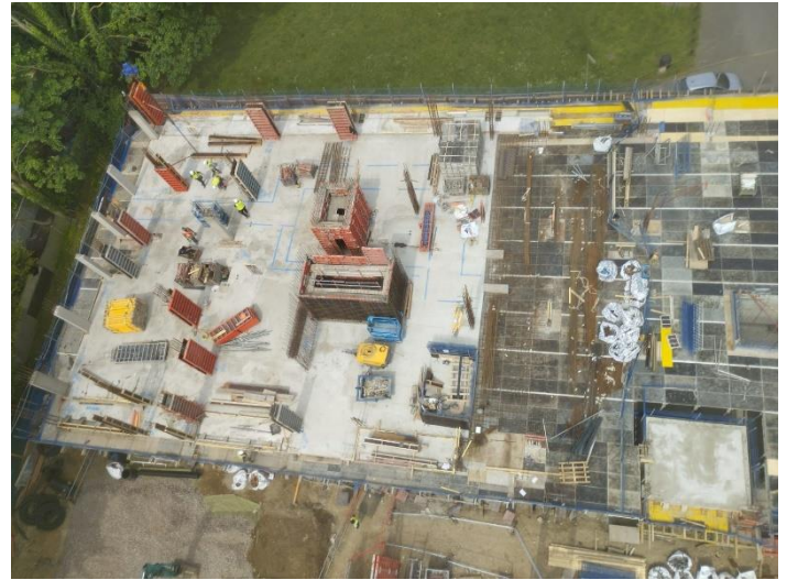
Overview of First Floor Core A
