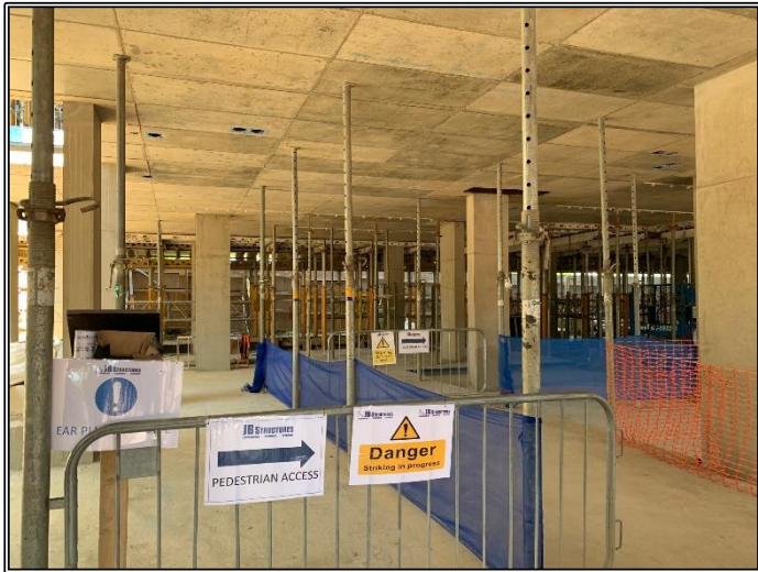
First Floor Formwork Removed
