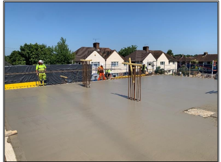
First Floor Slab Complete
