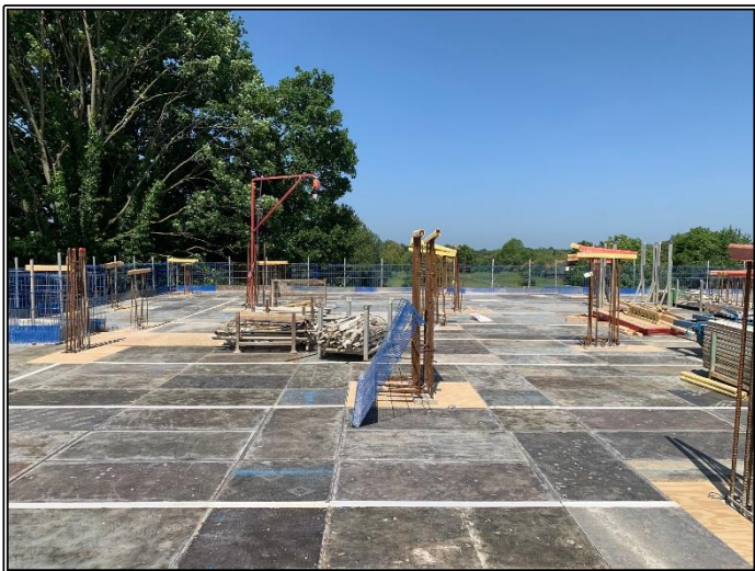
Second Floor Formwork
