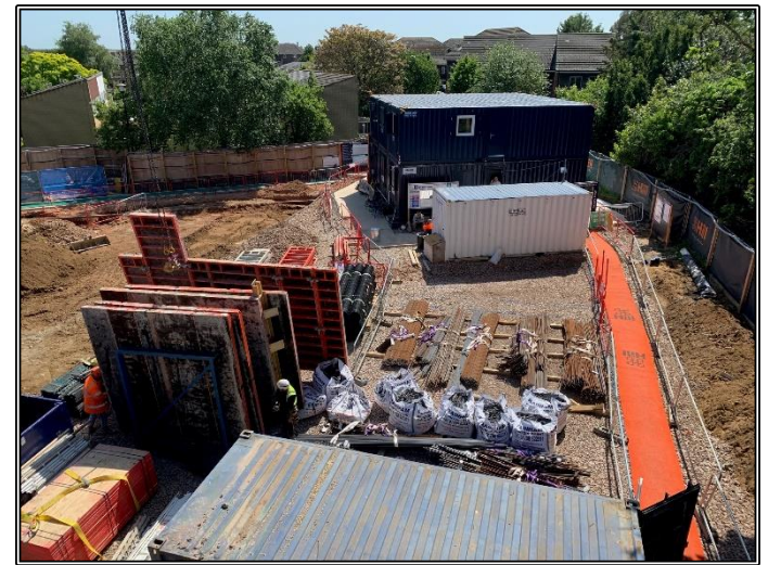
Site Compound, Walkway & Storage
