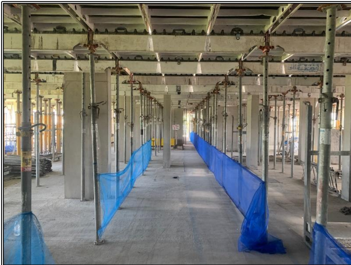
First Floor Slab
