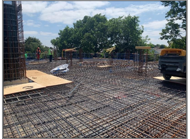
Second Floor Reinforcement
