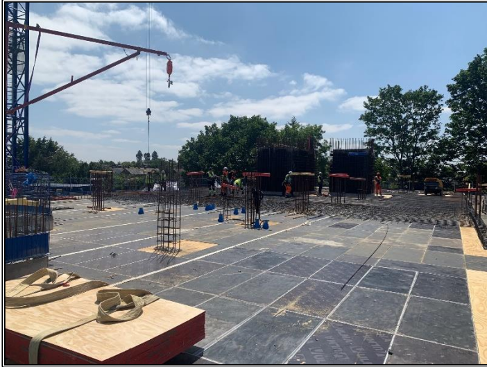
Second Floor Formwork
