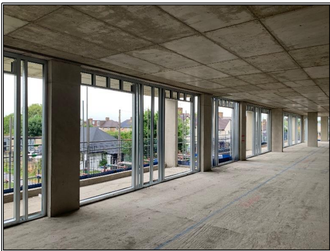
First Floor SFS In Progress
