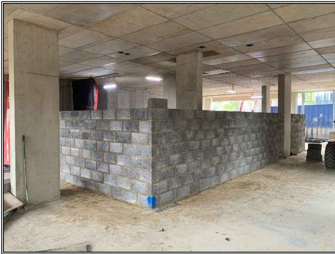
Ground Floor Blockwork
