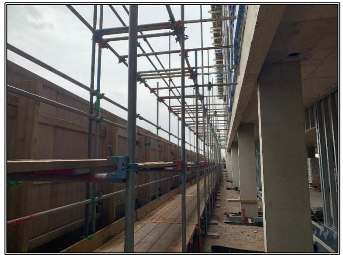
Scaffolding Has Commenced
