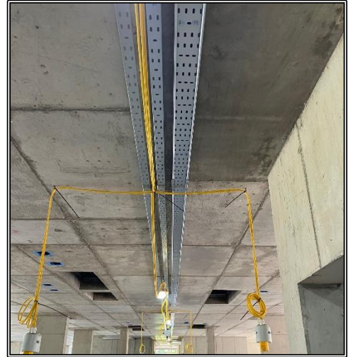
Electrical Containment Started
