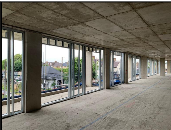
Second Floor SFS In Progress
