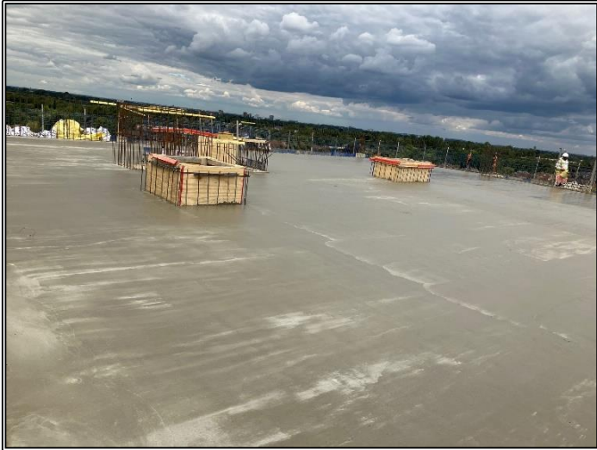
Core B Roof Slab
