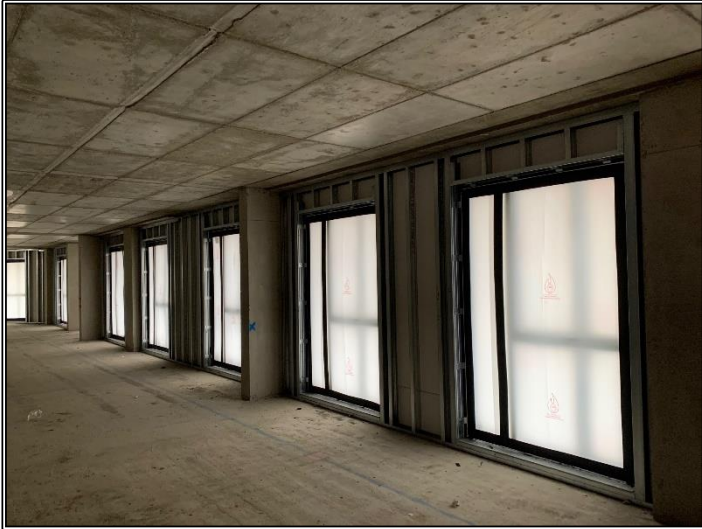
First Floor Windows Complete
