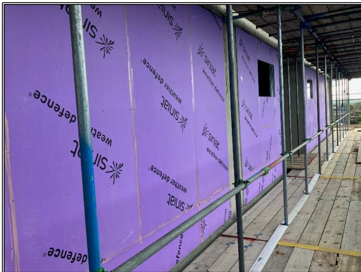
6 th Floor Boarding
