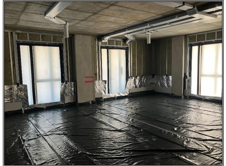
1 st Floor Screed Insulation
