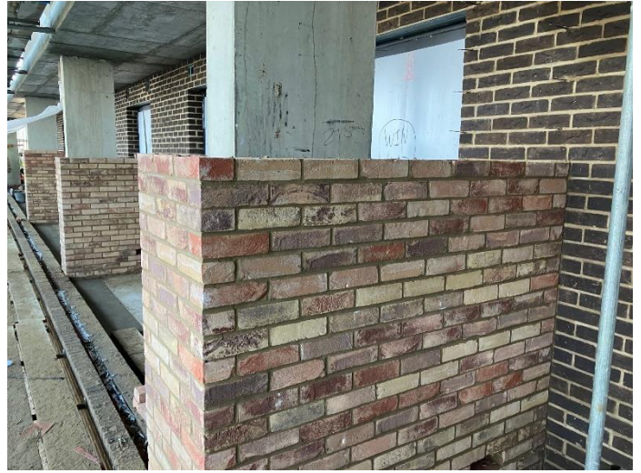
North-West Elevation Brickwork
