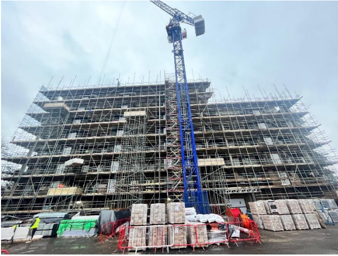
View of Building
