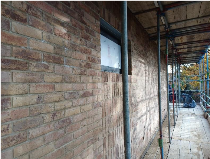
South-West Elevation Brickwork
