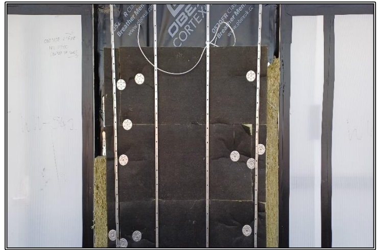
5 th Floor External Insulation
