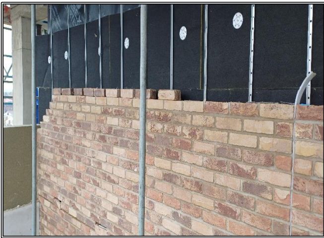
6 th Floor Roof Brickwork
