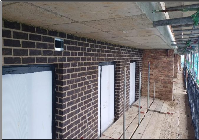
6 th Floor Brickwork Complete
