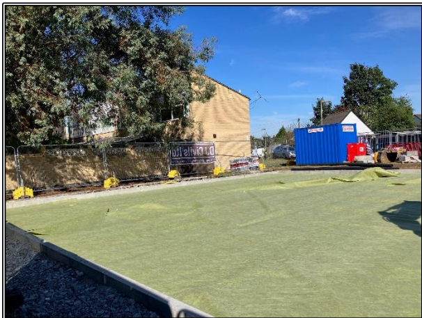
Car Park ready for Block Paving
