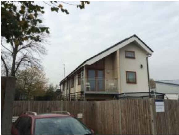
Mortlake Road, Richmond
