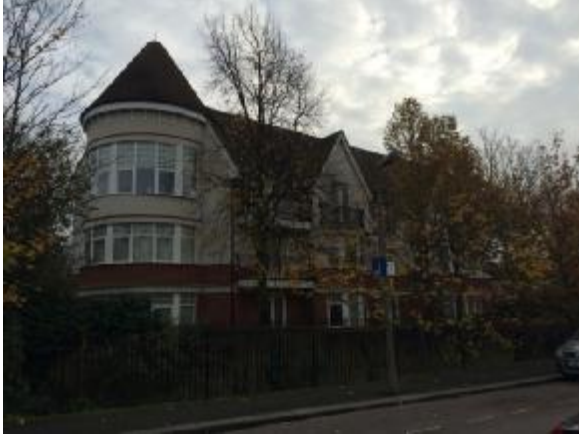
The Coterie Apartments, 16 Willow Av, Barnes
