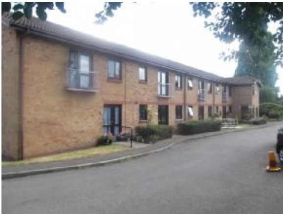
Paul Vanson Court, New Berry Lane, Hersham
