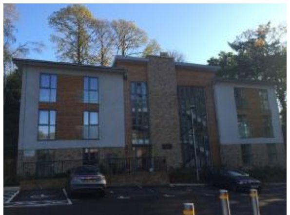
Lambert Court, Railton Close, Weybridge
