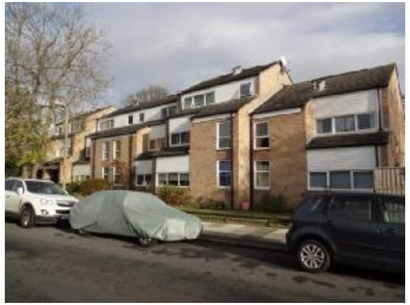
Trinity Court, Vicarage Road, Twickenham
