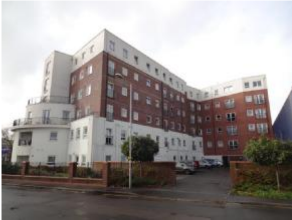
Crown House, 165 Kingston Road, New Malden
