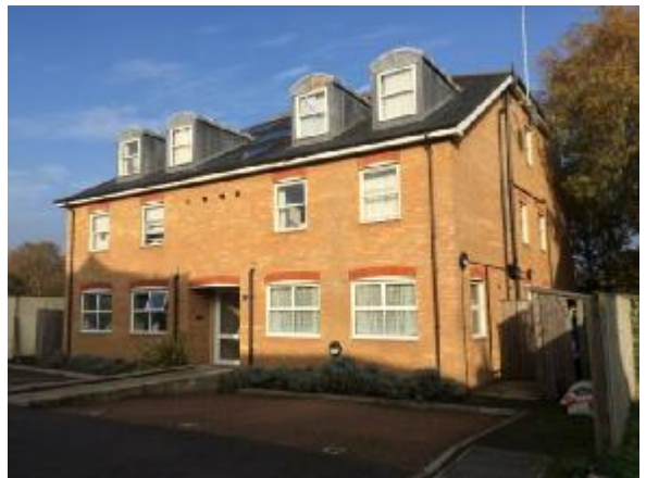
Rowntree House, Rowntree Road, Twickenham
